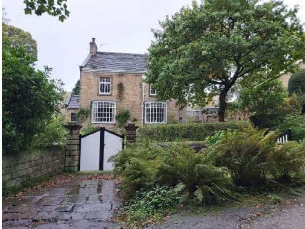
Insert 5-5 Dial House (HA6) seen from Old Hall Lane (looking northwest)
