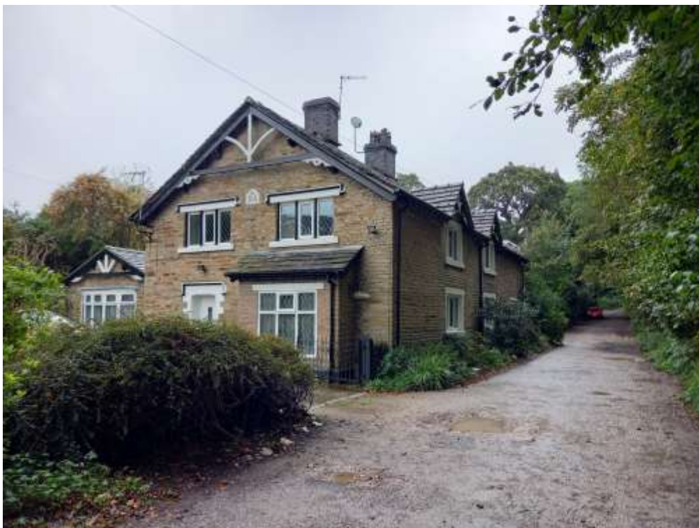
Insert 5-6 The Cottages north of Old Hall Lane (HA78) looking northeast
